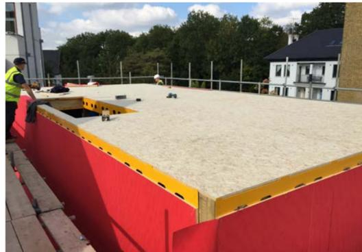
OSB fixed to floor joists
