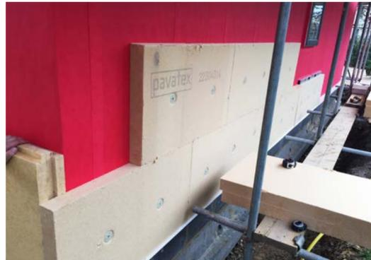
Breathable external insulation skin removes thermal bridges
